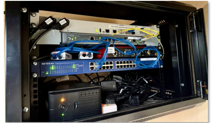
The final install at the caravan park
